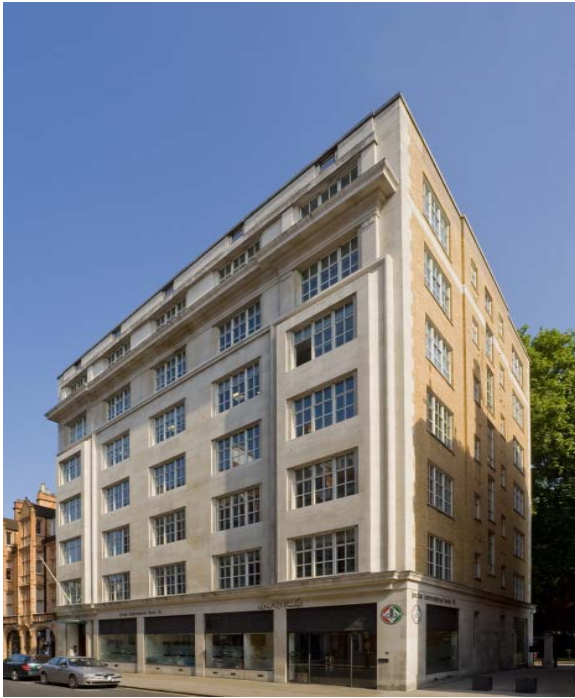
<Front of building>
